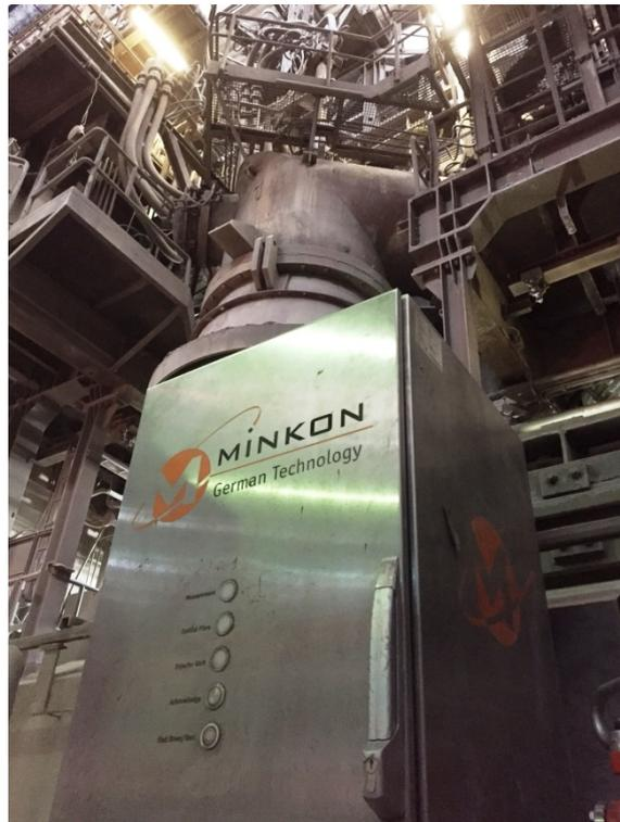
**Figure 1:** Photograph of the demonstrator for fibre optical temperature measurements installed at the vacuum degassing plant
