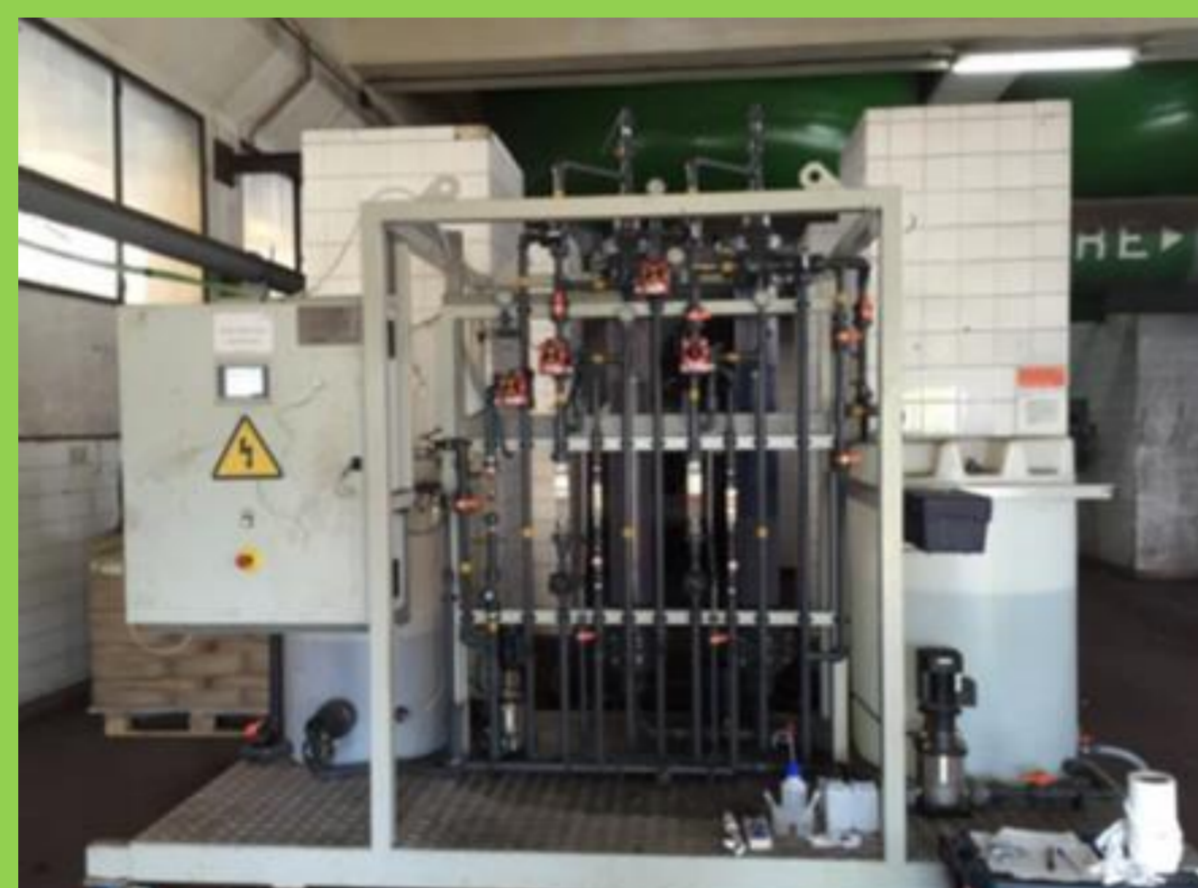
Filtration unit with 3-layer filter
