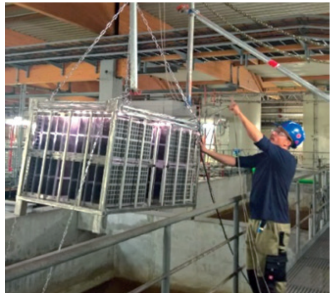
Figure 2: MOL ® LIK installation @ power plant
